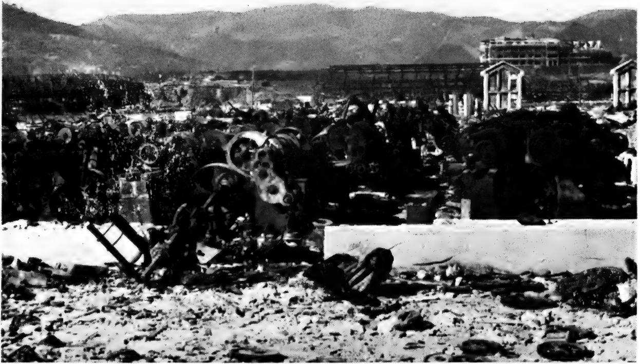
Photo No. 13. NAGASAKI. \frac{1}{2} mile from centre of damage. Typical damaged machines in one of the many timber workshops destroyed by blast and fire. Some machines were overturned by movement of the buildings, some destroyed by fire alone ; others damaged by exposure to the weather. See paragraph 34.
